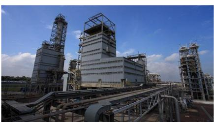
Existing PE plant in Cilegon with capacity 336 KTA where 1 train is UNIPOL PE Technology 200 KTA and another train 136 KTA is SDK
